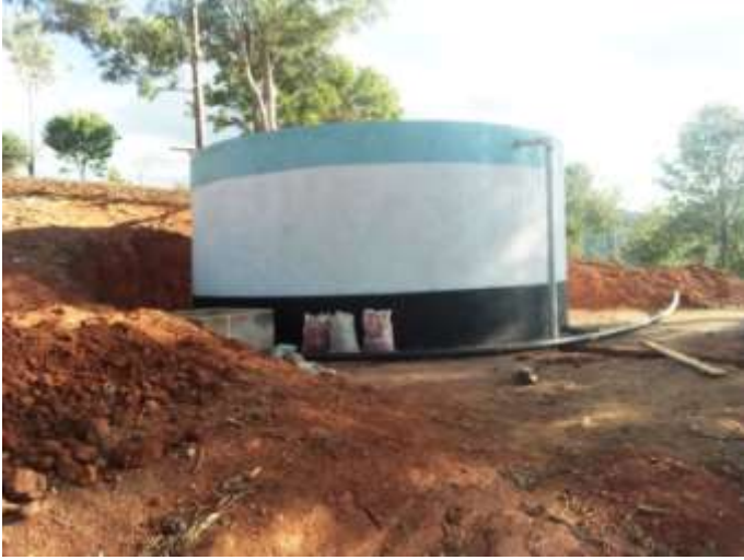
The 45m 3 storage tank for 9DPs at Kifuruga
