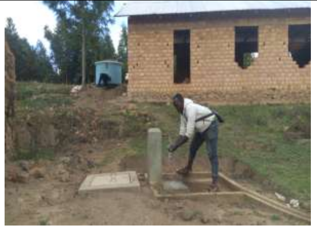
A water point (DP) at Pre-School (gets water from pipe network or from calabash tank (rain water))
